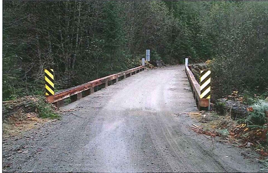
CK2141 Approach Right Bank
