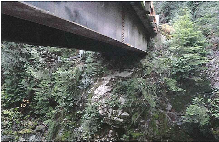
CK2141 Abutment Right Bank
