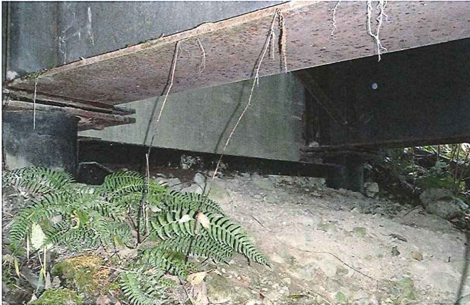
CK2141 Abutment Left Bank
