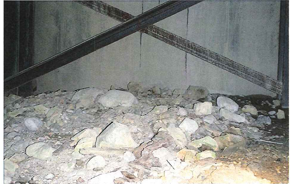
CK2141 Abumtment Right Bank #2
